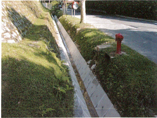
Channel Drain Installed at Merryn Road.
